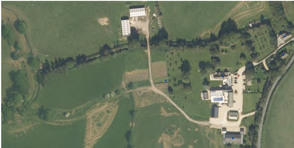
21 - Latest aerial photograph
